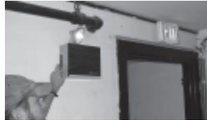
The emergency lights were also rewired and connected to the fire alarm
